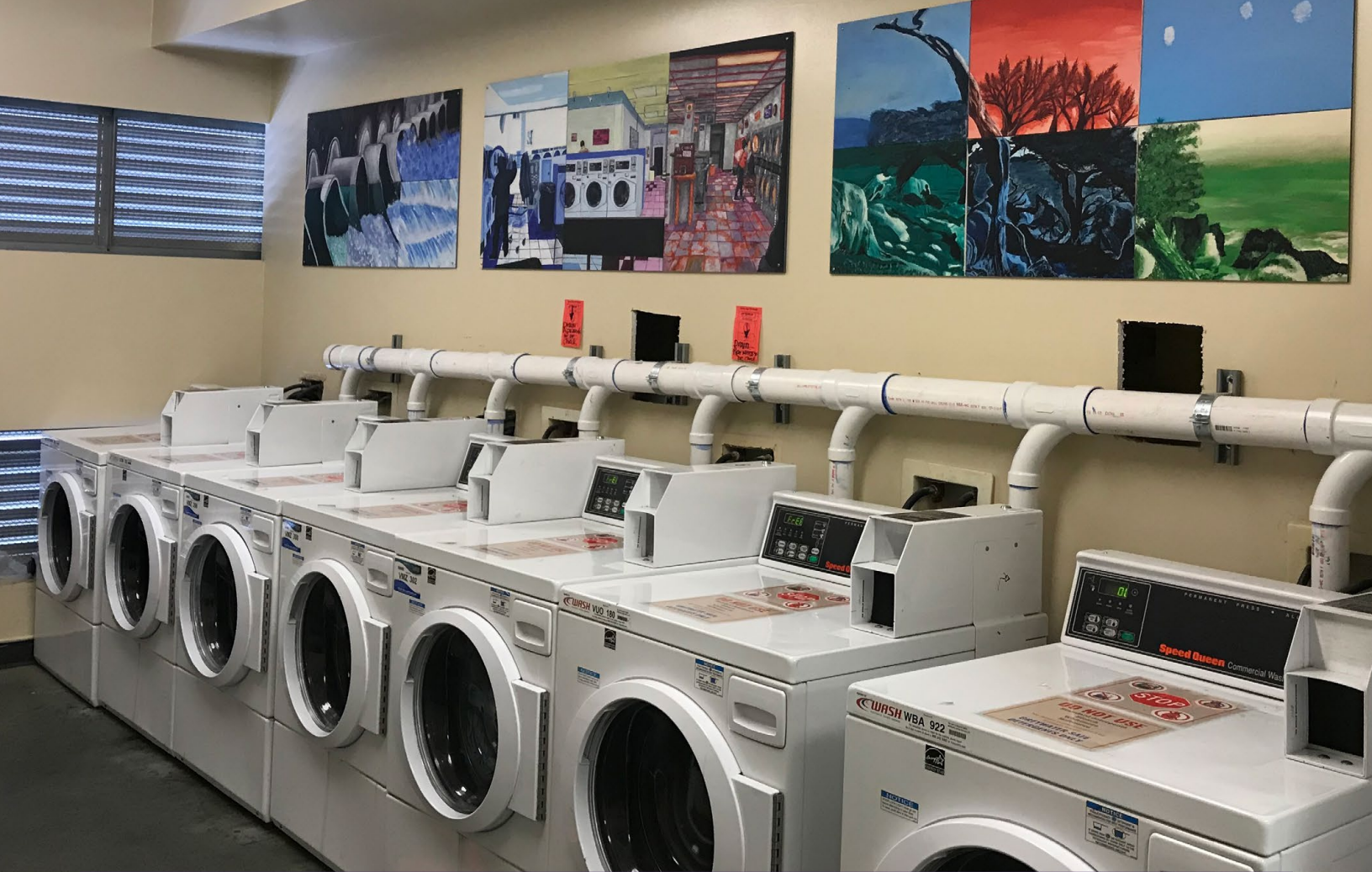
Laundry to landscape system installed in Pinnacles and features art developed by CSUMB faculty and students
