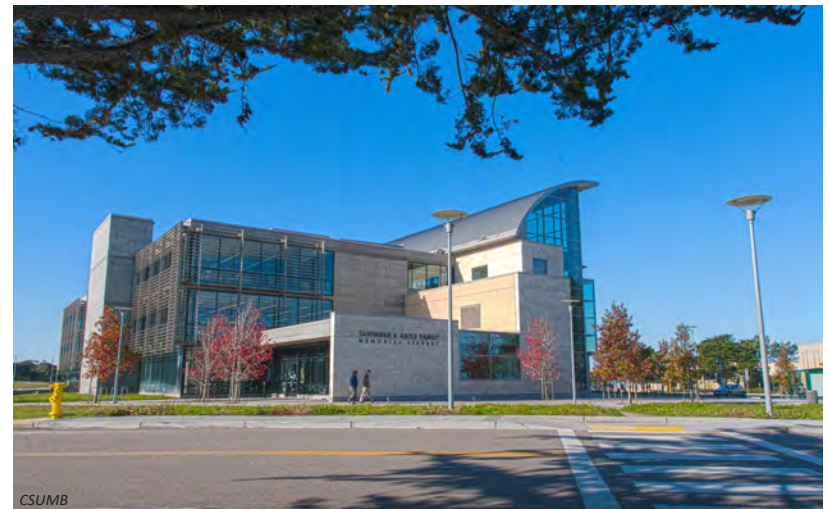
The Science and Academic Center (upper), and Library (lower) are two of the newer buildings on Campus, and are well-suited to the needs of students.
