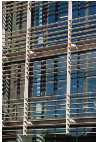
Building envelope, including the use of sun shades, modulates ventilation and solar gain.
