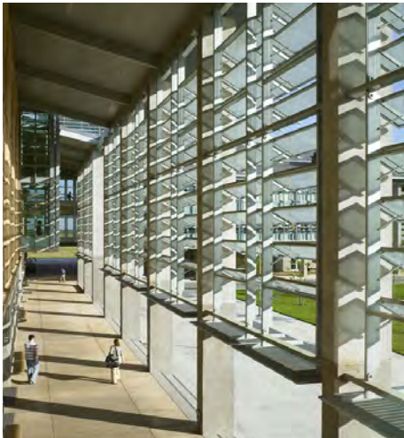
Building envelope, including the use of sun shades, modulates ventilation and solar gain.
