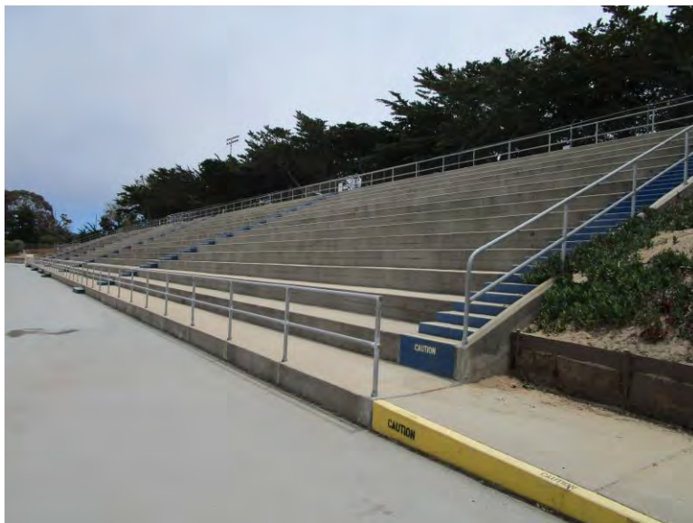
Figure 4. South bleachers, looking southeast (IMG_0434)
