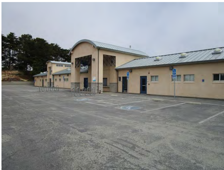
Figure 1. Main (west) elevation, looking northeast (IMG_0431)
