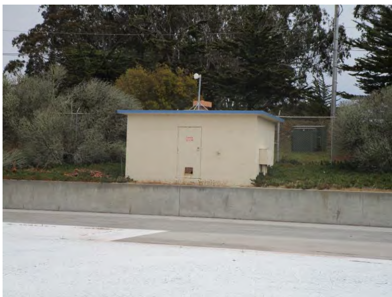
Figure 5. Electrical building, looking east (IMG_0452)
