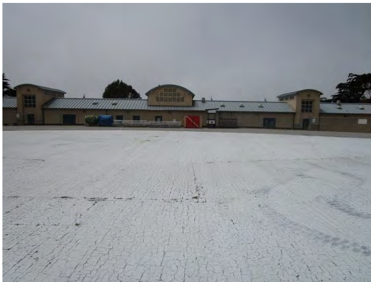
Figure 2. East elevation, looking west (IMG_0477)
