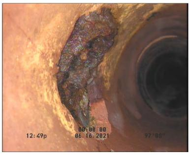
Photo: 4\_1\_5\_16062021\_150225\_A.JPG 97.64FT, Repair Patch, from 11 to 01 o'clock, within 8 inches of joint: YES
