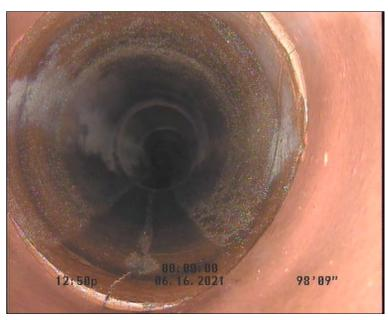
Photo: 4\_1\_6\_16062021\_150308\_A.JPG 98.74FT, Crack Circumferential, from 01 to 07 o'clock, within 8 inches of joint: YES
