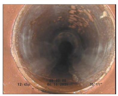
Photo: 4\_1\_3\_16062021\_145744\_A.JPG 35.88FT, Crack Circumferential, from 04 to 08 o'clock, within 8 inches of joint: YES
