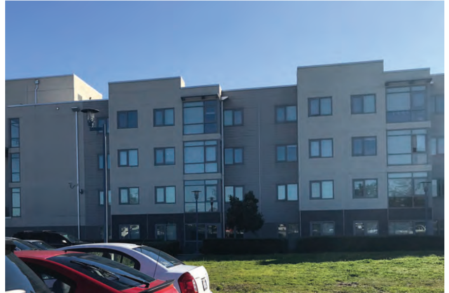
North Quad Housing (Main Campus)
