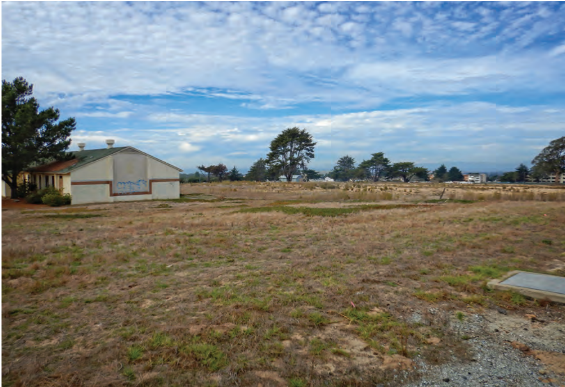
Abandoned former military building near Colonel Durham Street and 7th Avenue
